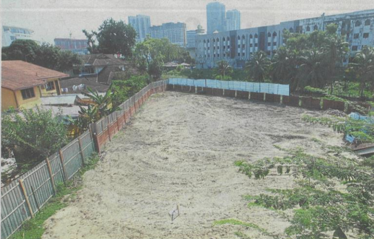
Two former bungalow plots in Section 14, Petaling Jaya, will now house a large building and residents fear it may be turned into a hostel.
